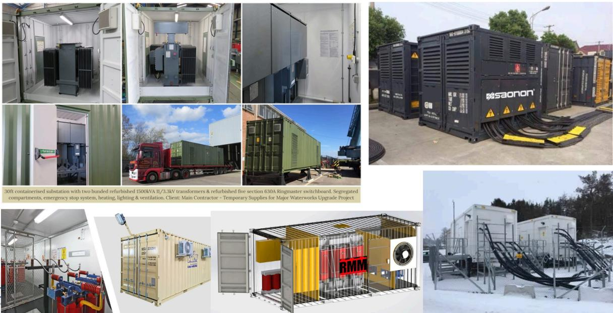
30ft containerised substation with two bunded refurbished 1500kVA 11/3.3kV transformers & refurbished five section 630A Ringmaster switchboard. Segregated compartments, emergency stop system, heating, lighting & ventilation. Client: Main Contractor - Temporary Supplies for Major Waterworks Upgrade Project
