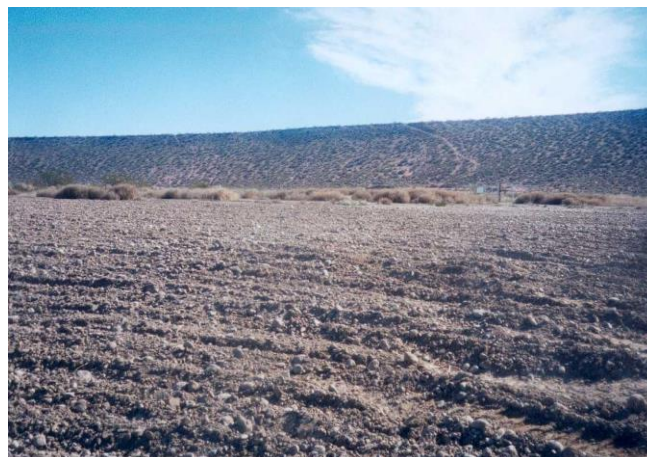
Figure 13. View of the ground after concluding the treatment.
