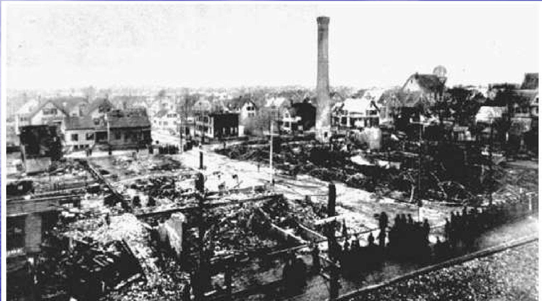
Figure 1.2 Shoe factory after the boiler explosion of March 20, 1905, which led to the adop-
