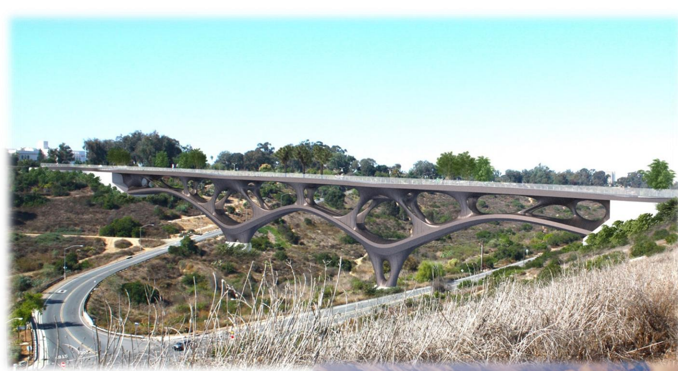
Puente peatonal en San Diego, California (3D steel printing)
