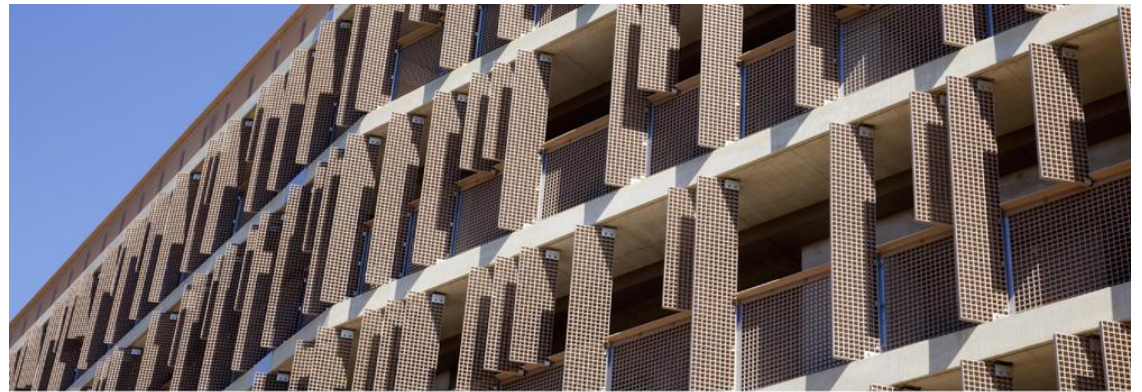
FIBERGLASS SCREEN DETAIL ON WEST BALCONY
