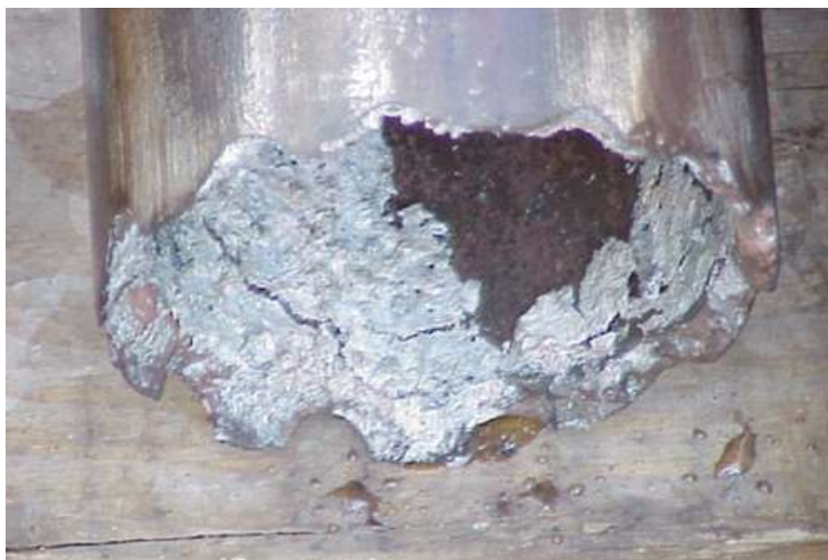
Fig. 4.16—Cut produced by a thermite cutter.
