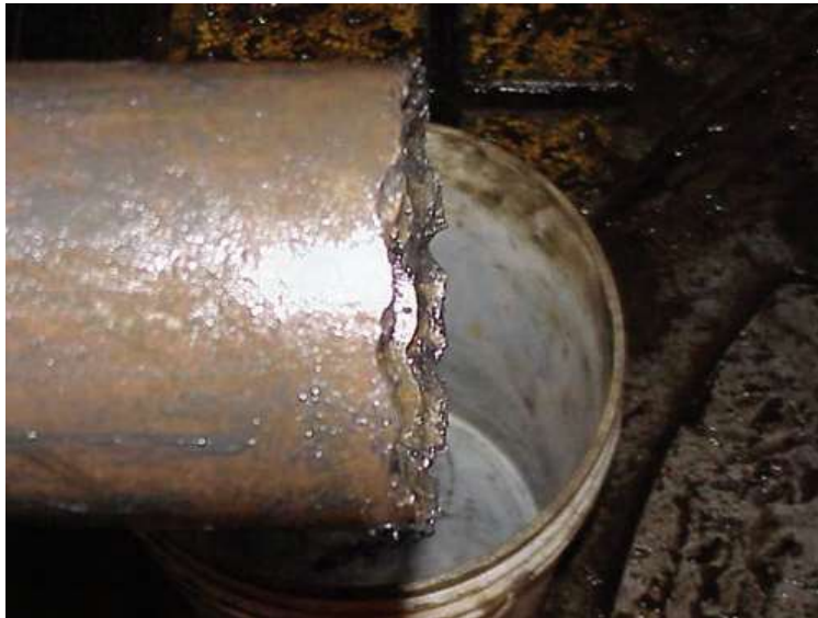
Fig. 4.14—Chemical cut pipe.
