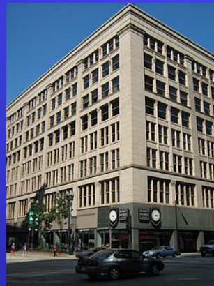
Second Leiter Building Le Baron Jenney (a+i) Chicago
