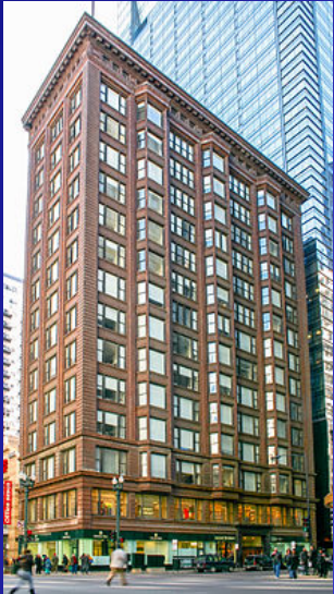
Chicago Building Holabird y Roche Chicago
