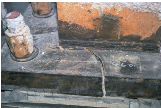
Fig. 1-22. Fractura en una placa de base de columna de una estructura de pórtico arriostrado (Earthquake Engineering Research Institute, Slides on the January 17, 1994, Northridge Earthquake, Set I: An Overview).
