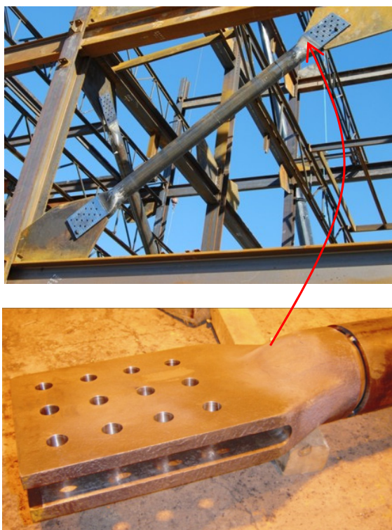
Figura 5-50. Conexión Cast ConneX High-Strength Connector ( http://www.castconnex.com ).
