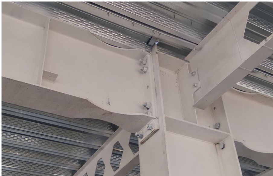
RBS (Reduced beam section) en vigas principales
