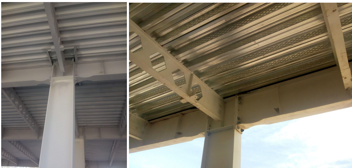
Figura 8: entrepisos Steel Deck
