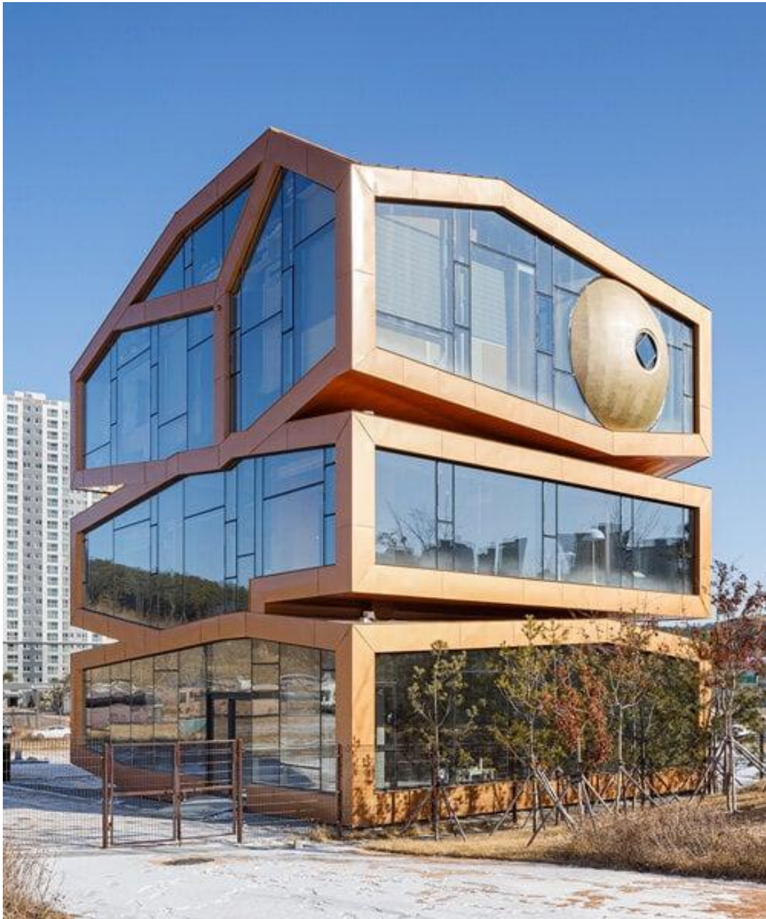
MARS building / Arq. Moon Hoon. /South Korea.
