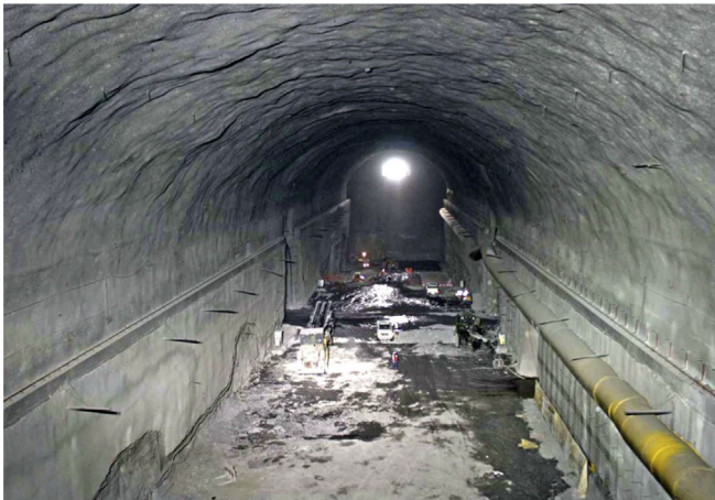
Fig. 24. The 26 m span, 50 m high Ingula underground powerhouse cavern after excavation of bench 3. Photograph provided by G. Keyter and reproduced with permission of ESKOM South Africa.
