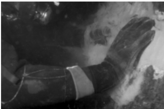
Fig. 6.2—Hand placing underwater patch. (Courtesy of M. Garlich.)
