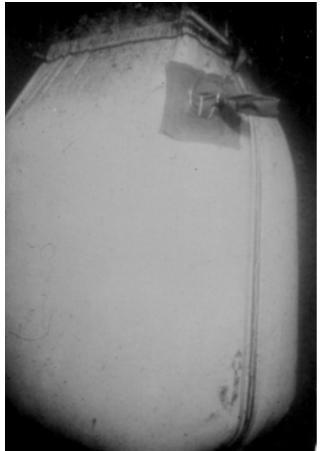
Fig. 5.5—Underwater view fabric form repair. (Courtesy of M. Garlich.)
