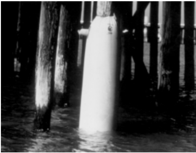
Fig. 5.6—Fabric form repair on timber pile. (Courtesy of M. Garlich.)
