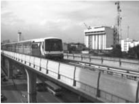
Fig. 5.16—Thin reinforced cementitious parapets used on the BTS Skytrain in Bangkok, Thailand.
