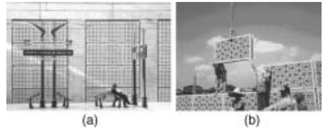
Fig. 5.14—(a) Use of thin reinforced cementitious acoustical wall panels at the TGV railway station, Charles de Gaulle International Airport, Paris; and (b) thin reinforced cementitious noise barriers.
