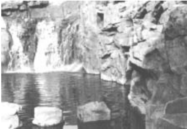
Fig. 5.17—Architectural rocks made using thin glass fiber-reinforced concrete.
