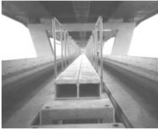
Fig. 5.9—Application of thin reinforced cementitious cable duct under a railway bridge.
