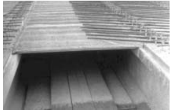
Fig. 5.15—Thin reinforced cementitious permanent formwork panels.
