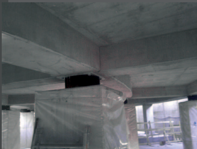
• L'AQUILA, ITALY - ANAS new Head Office: installation
