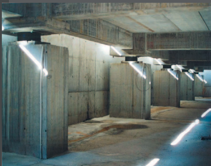
UDINE, ITALY - "Gervasutta" Hospital: installation
