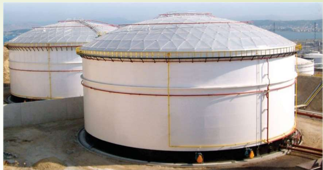
Techo flotante interior
