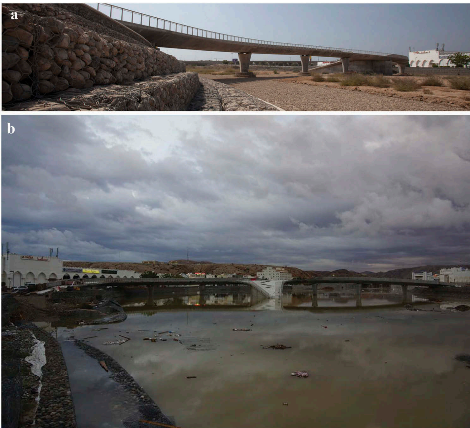
Figure 7. Top image, Wadi Adai in its dry state [image courtesy of Batco Engineering group, Copyright 2017 by Batco Engineering Group, reprinted with permission, retrieved from http://www.batco-group.com , (accessed 3 July 2018)]; bottom image showing the wadi in its wet phase and the flooded construction site; the upper stepped terraces can still be used in wet conditions. [Source: Courtesy of Snøhetta, Copyright 2013 provided by Kent Horne, reprinted with permission].
