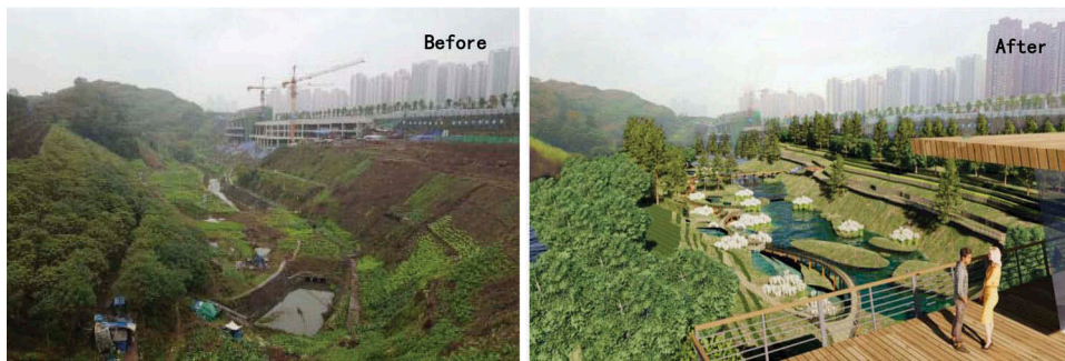
Figure 9. Before and after the reconstruction of Kangzhuang river in the midstream of the Tiaodun river.
